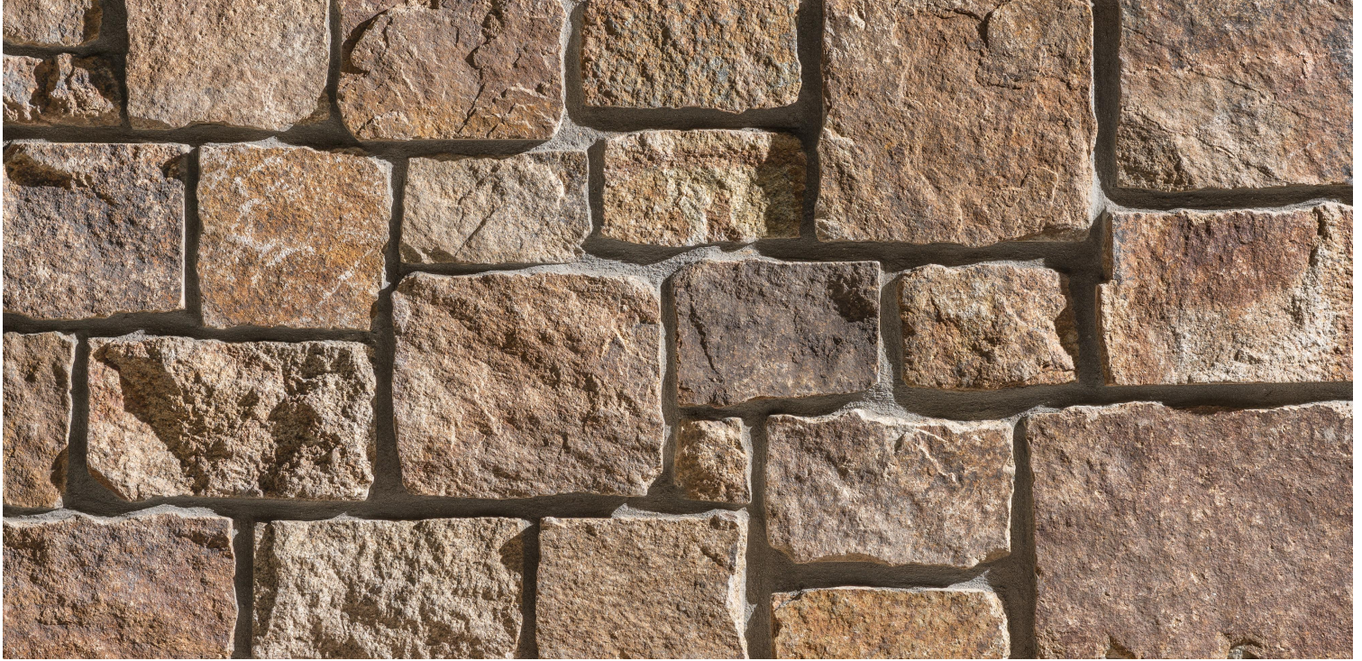
Photo Shows Installation With Mortar Joint
